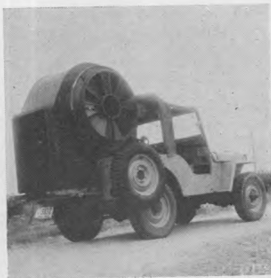
Fig. 16. The Universal jeep used as a truck to haul a large fan weighing about 725 pounds.
