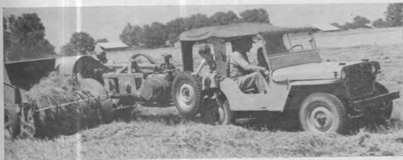
Fig. 11. The Universal jeep pulling a small pick-up hay baler. A total of 100 bales of hay were baled in one hour.
