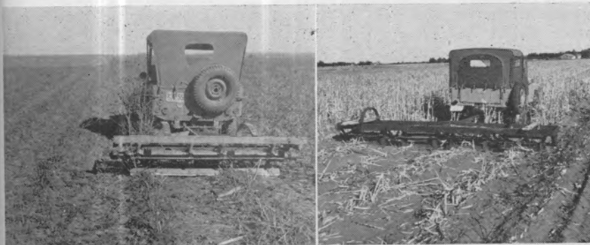
Fig. 3. Left—Military jeep pulling a two-row tractor type stalk cutter cutting cotton stalks. The cutter is hitched to the left end of the drawbar and the left wheels of the jeep are almost running on the row of stalks. Right—The Universal jeep pulling a four-row homemade stalk cutter cutting sorghum stubble. The cutter is hitched to the center of the drawbar of the jeep, thus making it necessary to drive with the wheels running directly on the two center rows.
